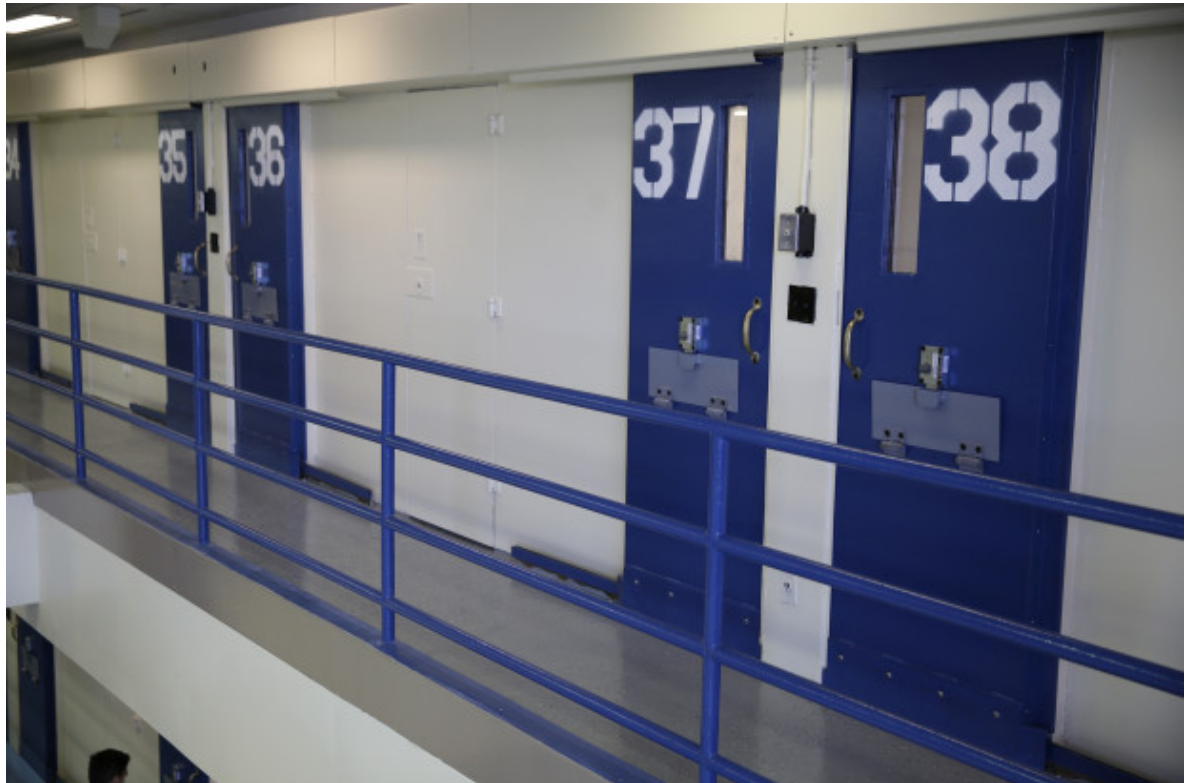
An enhanced supervision housing unit on Rikers Island. AP
